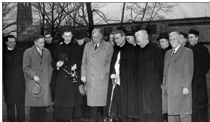
President John J. Long, S.J. (holding shovel), breaks ground for the Fieldhouse on December 8, 1947. Alumni Memorial Fieldhouse would go on to provide 59 years of memories for Saint Joseph's basketball.
